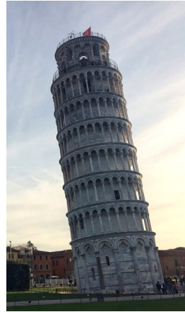
Leaning Tower of Pisa
